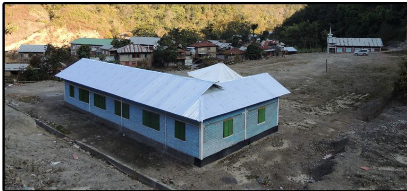
Lungthul (T) PCI School Building thak
